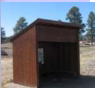
Bus stop Kiosk and Bulletin Boards
